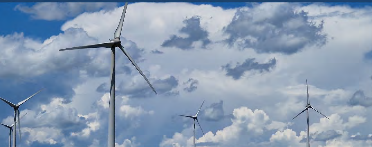
Premier Energy's 80 MW Wind Park, near Mihai Viteazu, Constanta County, Romania
