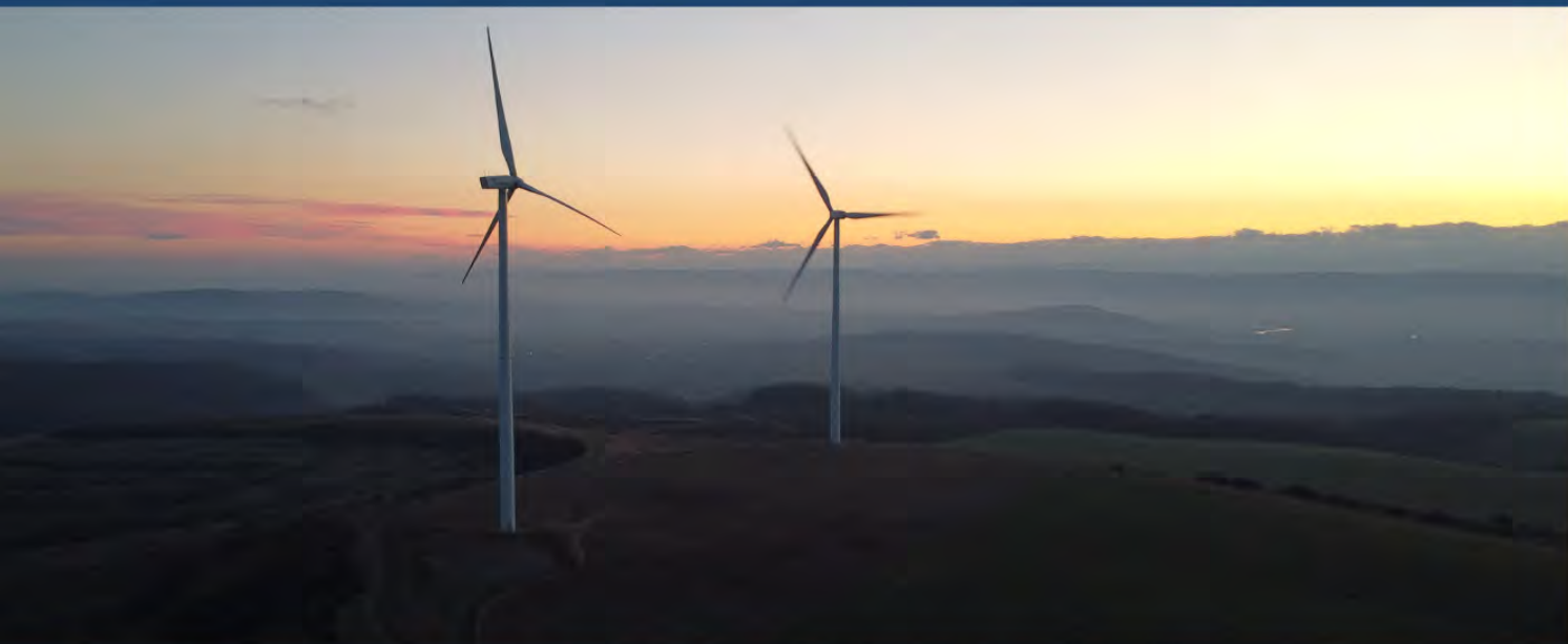
Premier Energy's 18 MW Wind Park, near Dranceni, Vaslui County, Romania
